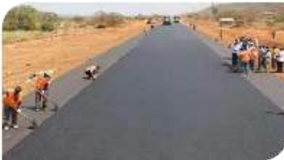
Figure 22: Construction of the Kibwezi- Mutomo- Kitui Highway
