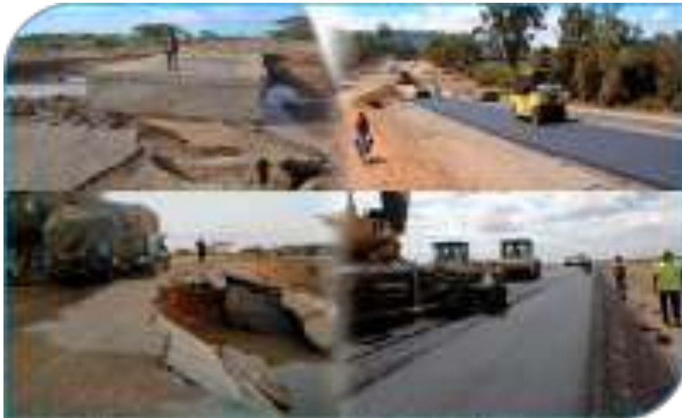
Figure 21: Rehabilitation of key infrastructure
